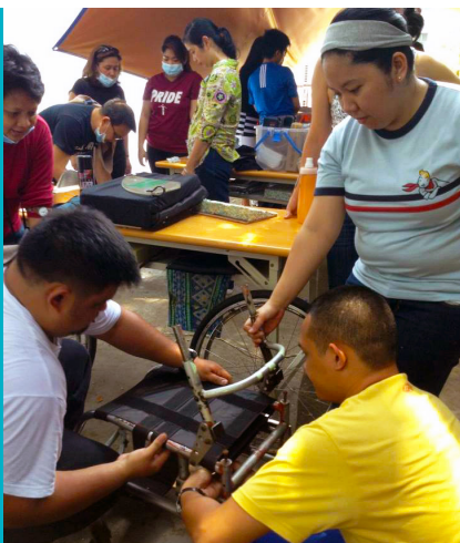
Program staff make adjustments on the wheelchair based on the user's needs and condition.
